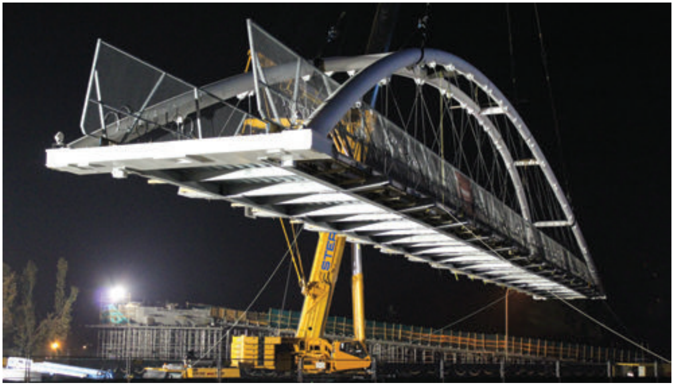
The Salton Road cycle and pedestrian bridge, built to exacting standards, is lifted into place by a 550-tonne crane as the Trans-Canada Highway 1 was shut down to accommodate the bridge's placement.
